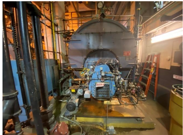
Dual natural gas/oil boiler
