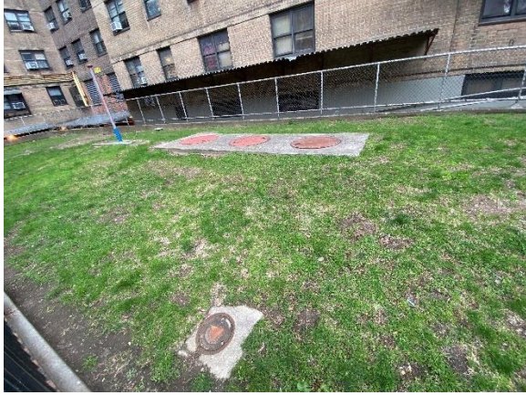
Vent pipe / UST and associated monitoring wells west of Building Chelsea - 1
