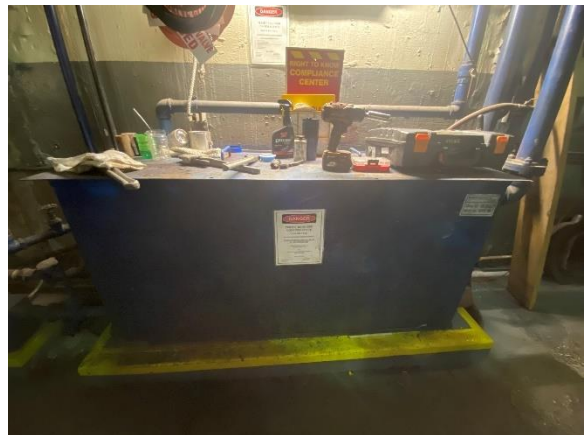
Holding tank – oil recovery/remediation system
